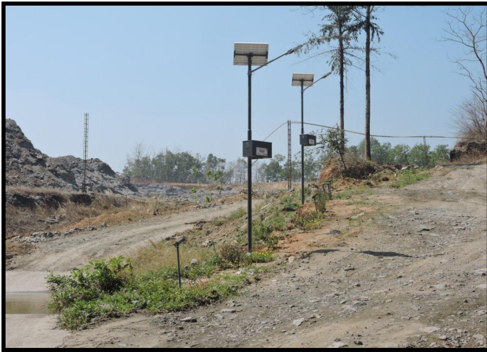
Solar light in the project site
