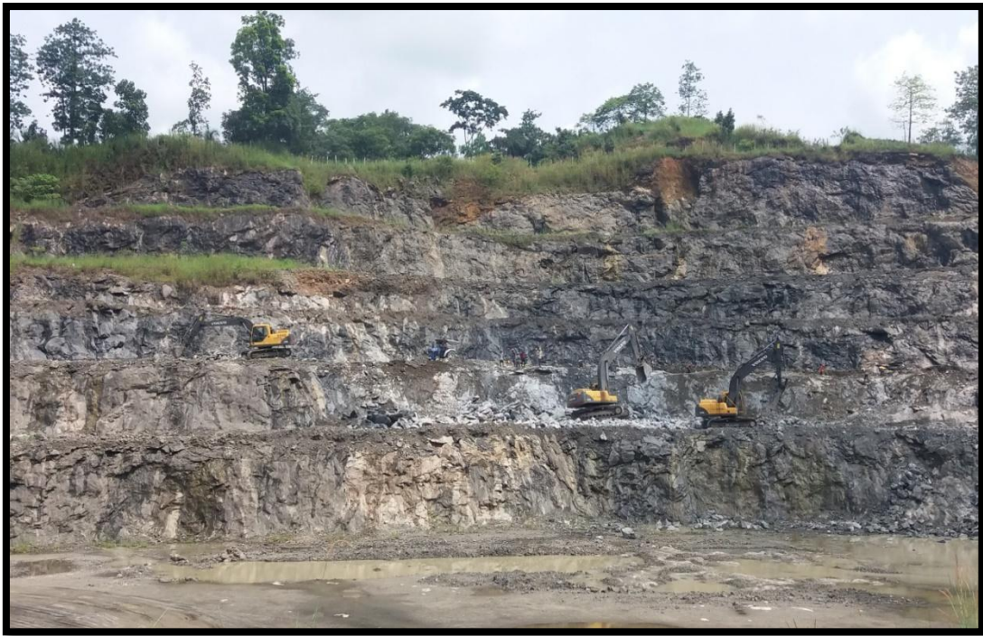
Photograph of benches created in the quarry site
