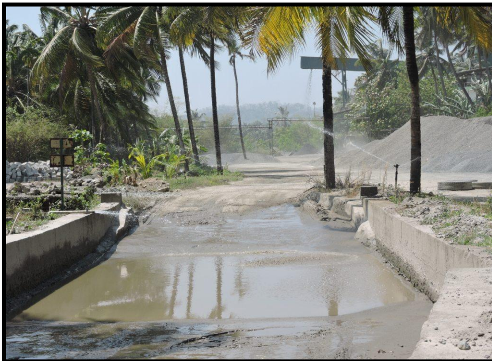
Sprinkler installed in project site
