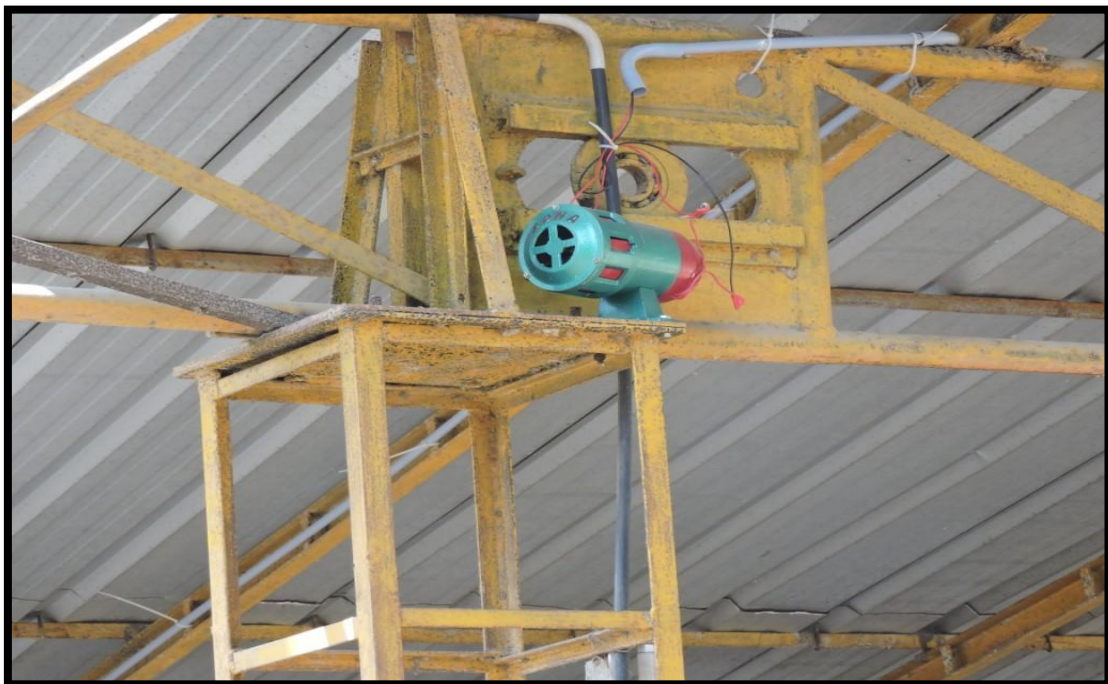
Warning alarm installed in the project site
