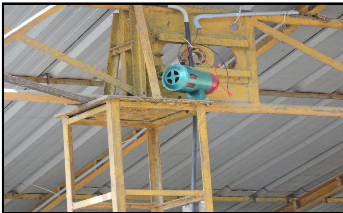
Warning alarm installed in the project site
