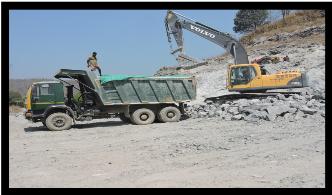
A covered truck; before leaving from the project site
