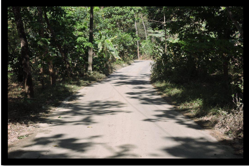
Tarred access road to the quarry site
