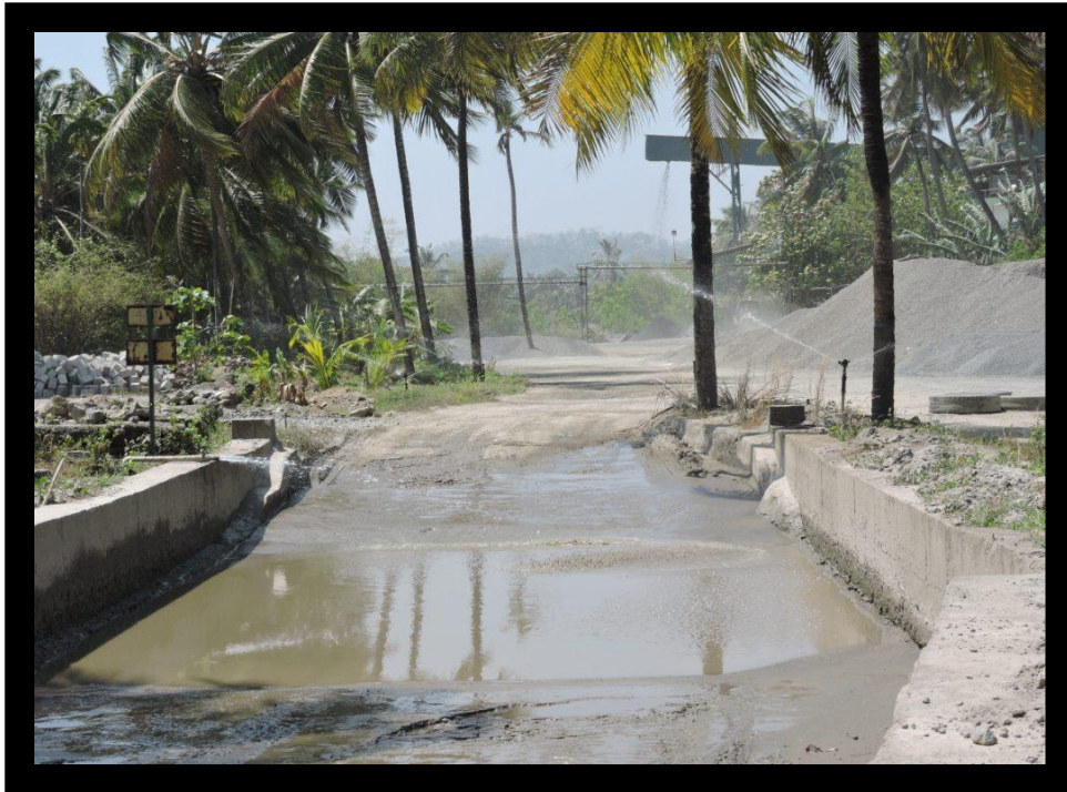
Sprinkler installed in project site
