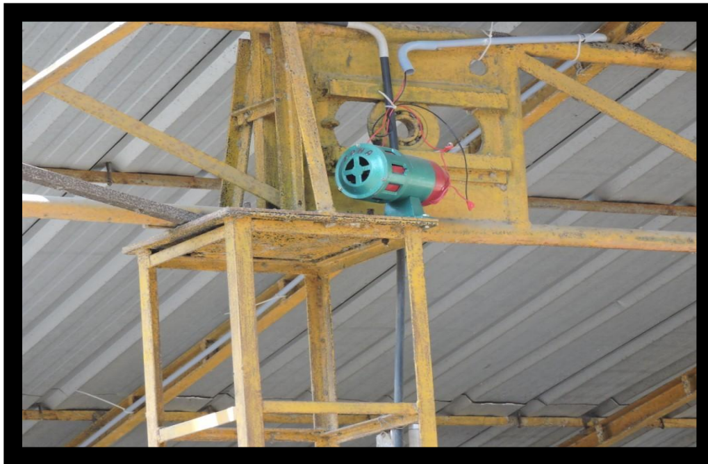
Warning alarm installed in the project site
