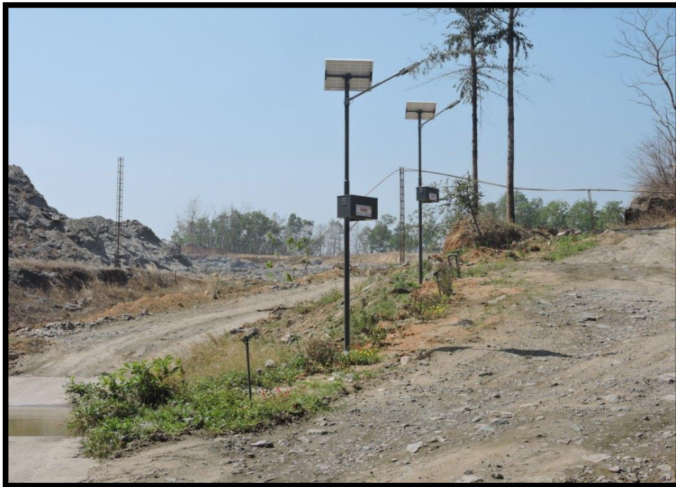
Solar light in the project site
