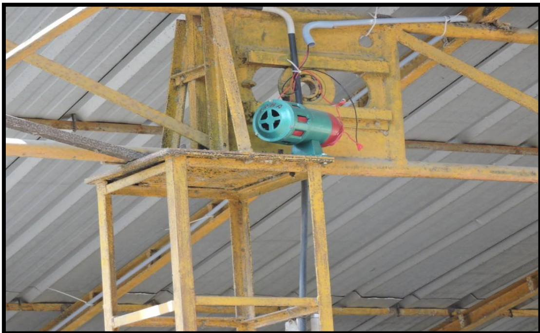
Warning alarm installed in the project site
