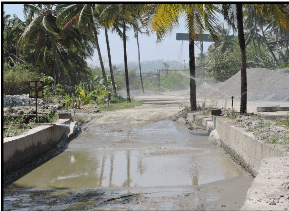
Sprinkler installed in project site
