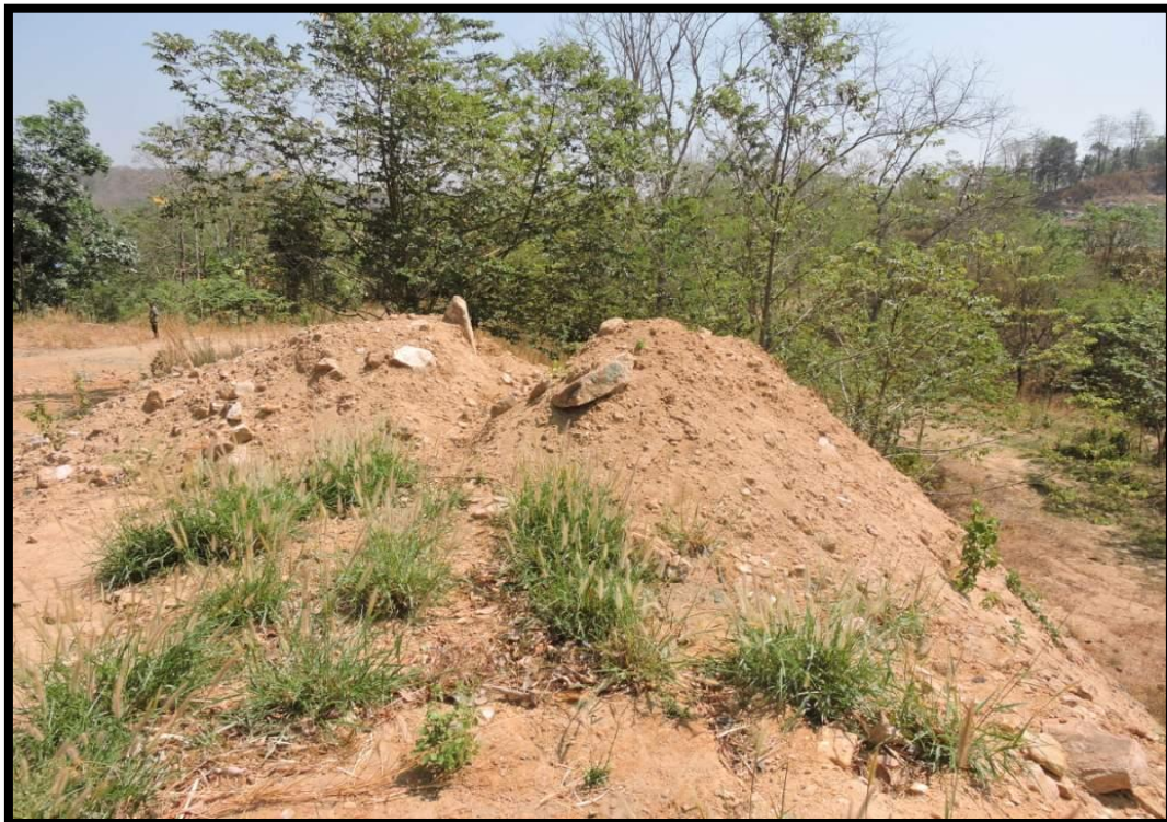
Overburden stacked in the project site.
