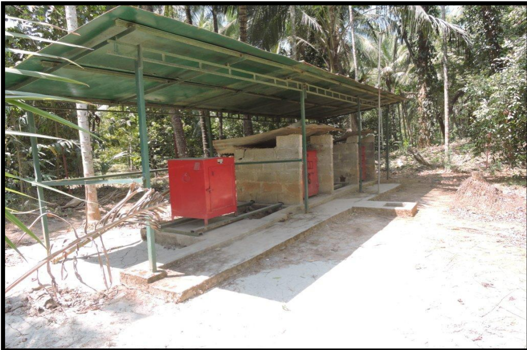
Magazines at isolated place in the project site
