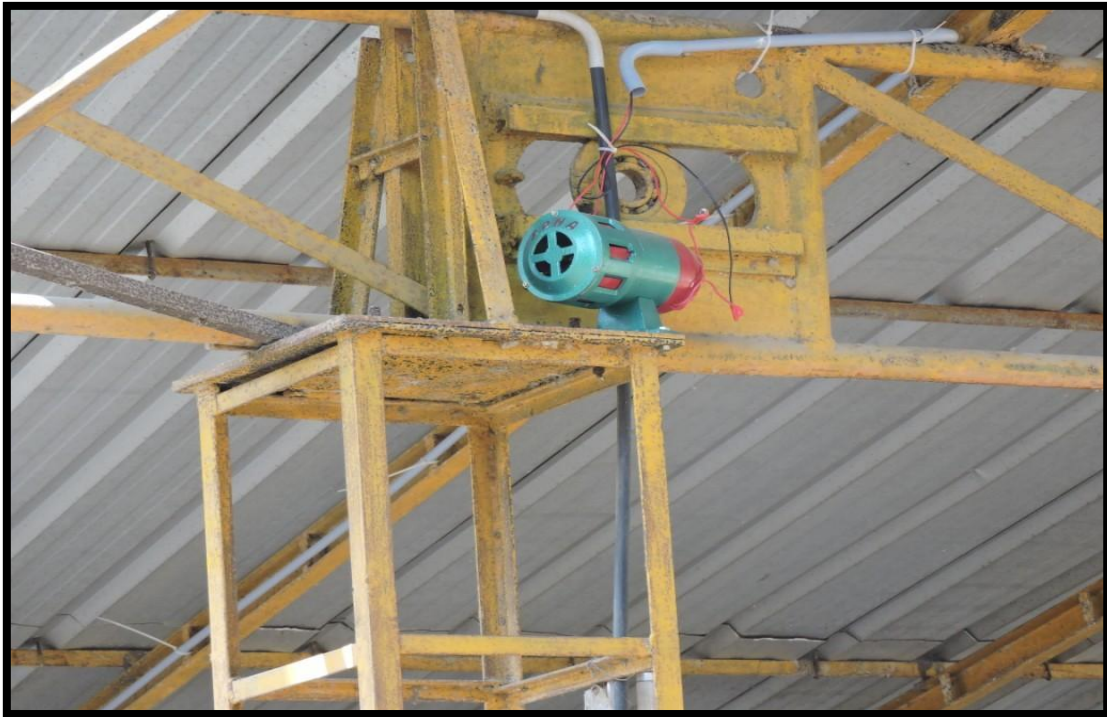
Warning alarm installed in the project site
