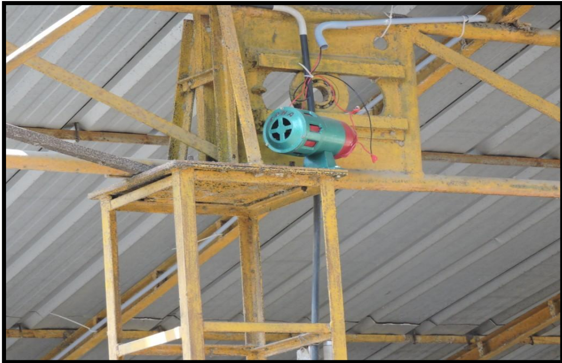
Warning alarm installed in the project site
